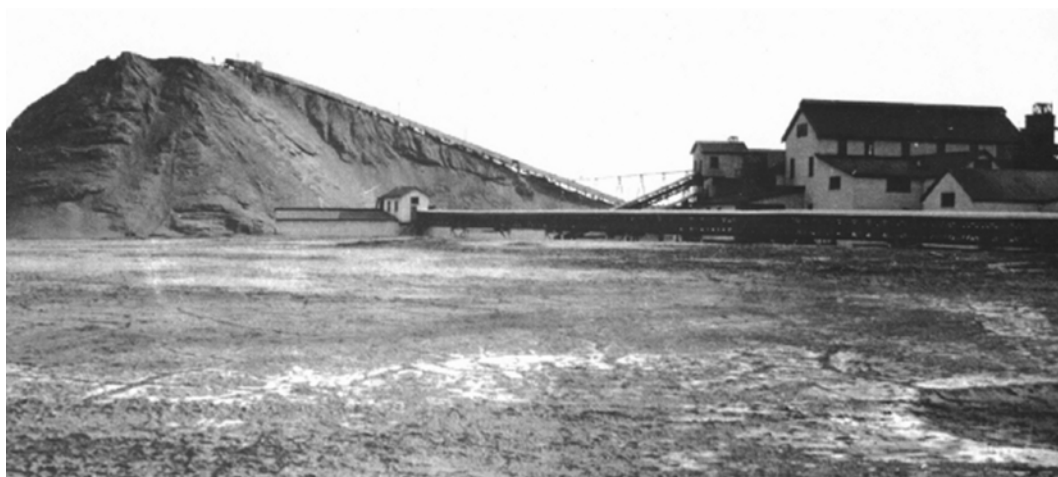
The Devon Mine showing the tailings dump, with picking tables housed in building at right.
